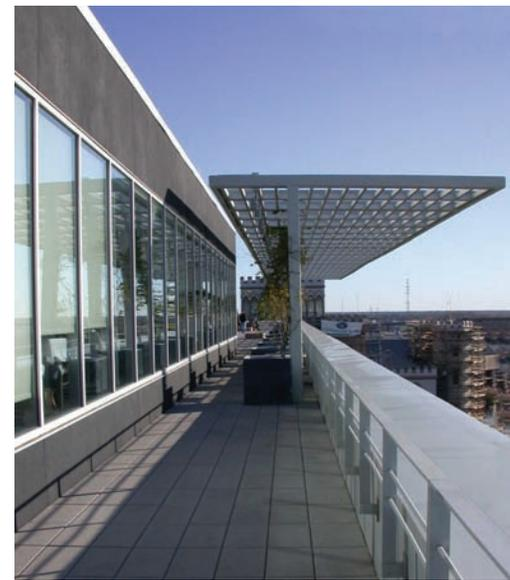
*Example of Solar Shading.*
